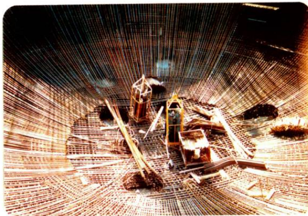
Figur 6. Armering undre kuleskall
