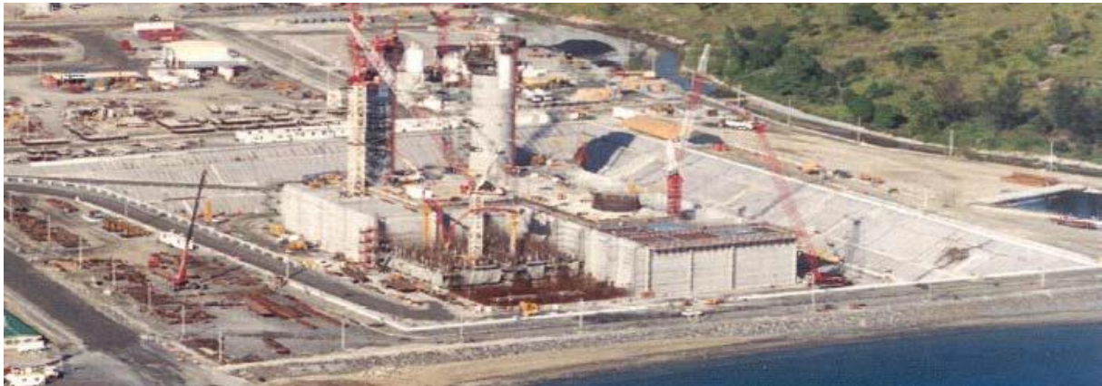
Figur 11 “Purpose built” tørrdokk [13].
