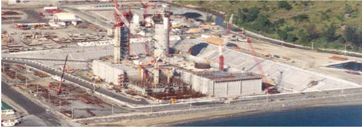
Figure 11 “Purpose built” dry dock [13].
