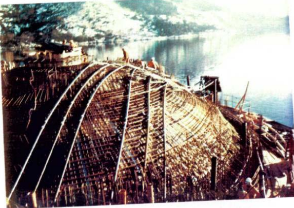
Figure 9 Reinforcement upper domes [13].
